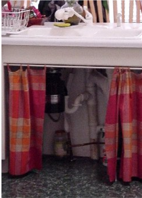
When doors under the sink are removed to create clear knee space, a curtain can be used to hide this area.
