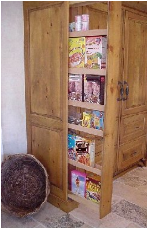
Narrow full extension shelves make it easy to reach items such as cereal boxes.
