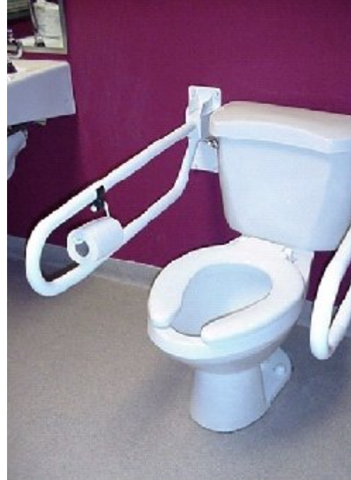
There are many types of grab bars for the toilet. Fold down grab bars can be used when the toilet is not by a wall or not by a wall that can be reinforced. Grab bars need to be reinforced so they can support 250 pounds of pressure. Placement of the toilet is important depending on the type of transfer someone must perform.
