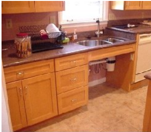
Lowering the counter top/sink height and clearing knee space underneath can make it easier for a wheelchair user. Lever controls for the faucet are easier to use for someone with impaired hand function. Raising the dishwasher puts it at an easier to reach height for someone standing and someone in a wheelchair.
